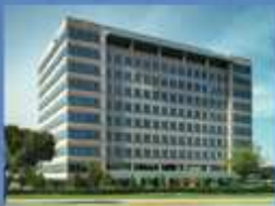
Granite Tower Dallas
