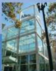
AboveNet Data Center Silicon Valley
