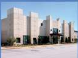
AT&T Web Hosting Facility Atlanta
