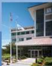
Converse Technology Bldg Boston
