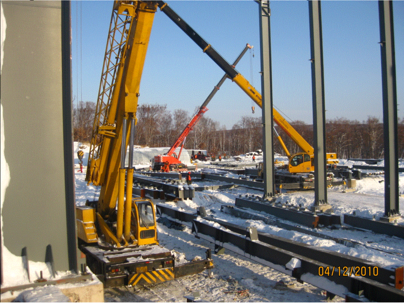
Figure 2: Construction at Eastern Dragon Project
