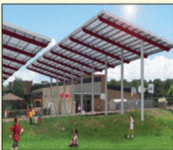
Schools & Government 7 MW completed + 6 MW in progress
